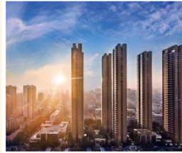
Shenyang Arcadia Court
