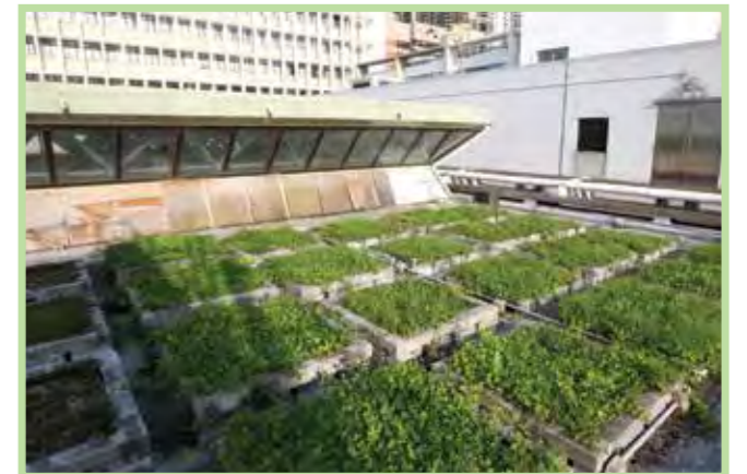
A green roof is set up at the University of Hong Kong, aiming to lower the temperature of the building and save energy. 香港大學設有綠色天台，能有效降低校舍室溫，節省能源。
