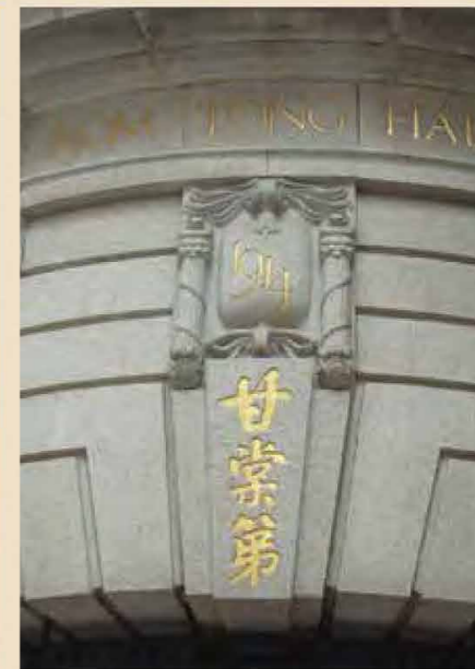
(Top left) With its arched facade, the former marine police headquarters in Tai O is a model of East-meets-West architectural elegance.
