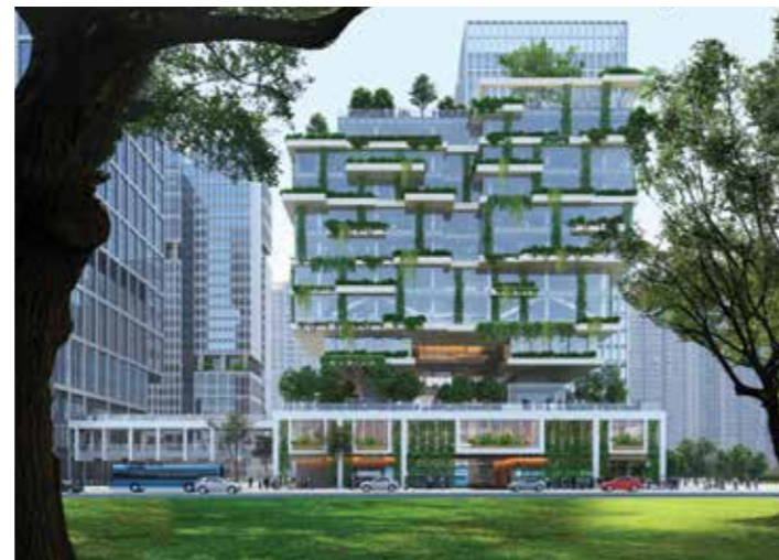
Biophilic design has been applied on various buildings under Kerry Properties' portfolio 嘉里建設旗下的多項建築均沿用「親和自然」的設計
