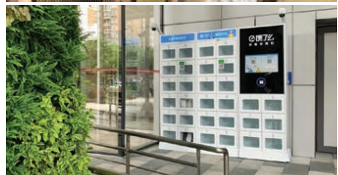
Contactless installation, Kerry Everbright City, Shanghai
