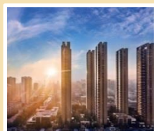
Shenyang Arcadia Court
