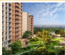
Nanjing Arcadia Court
